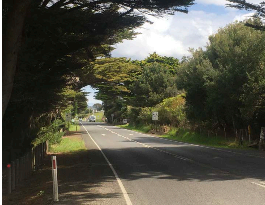
Figure 7-4 Viewpoint No.3 - Great Ocean Road east of Old Cable Station Museum
