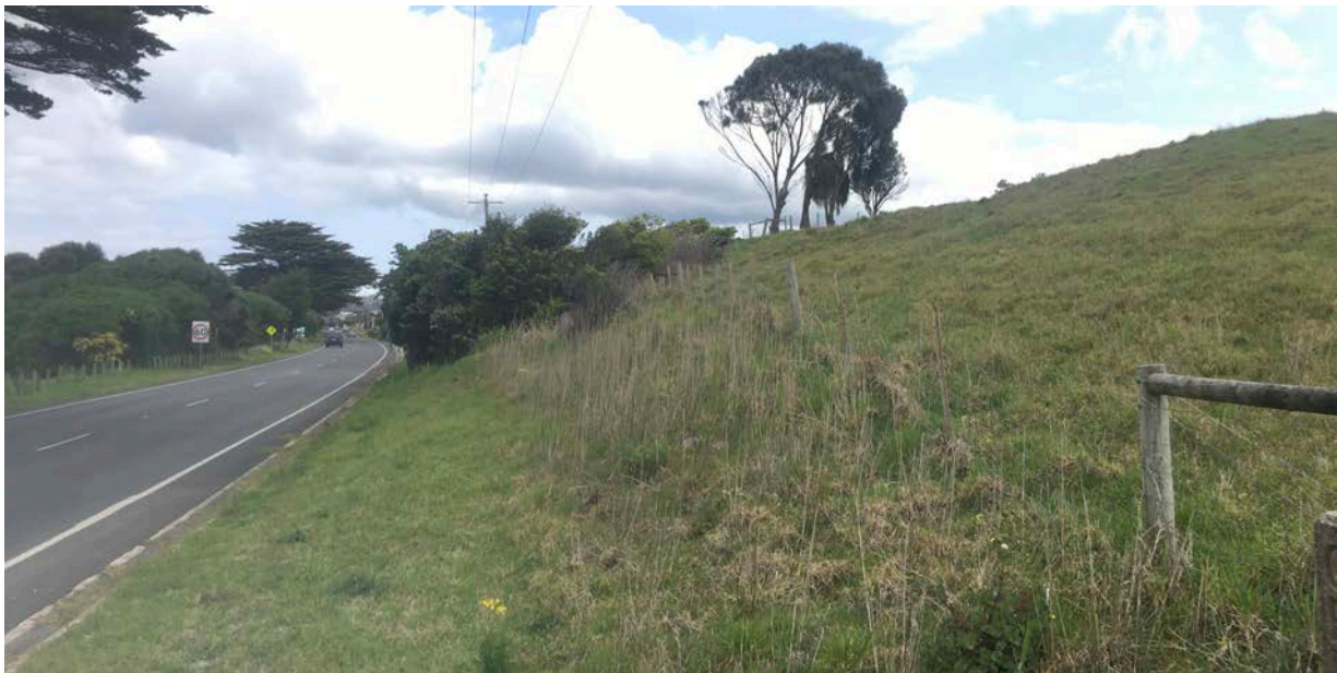
Figure 5-1 Steep grassed embankment to frontage of 6280 Great Ocean Road
