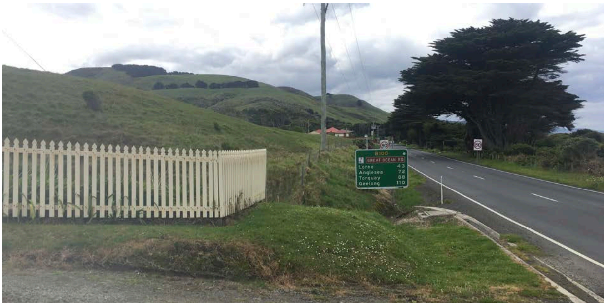
Figure 5-2 Grassed embankment to frontage of 6280 Great Ocean Road
