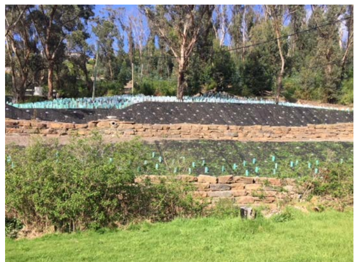
New Indigenous plants on the lower and upper embankment
