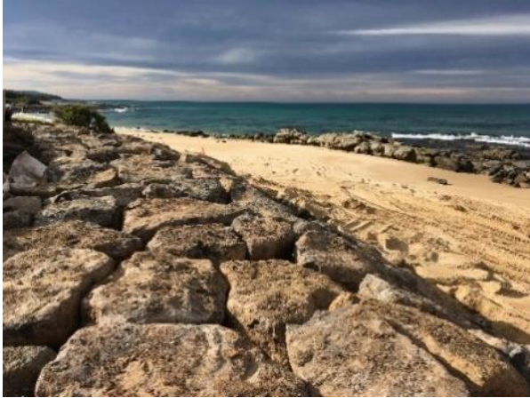
The new rock armour wall
