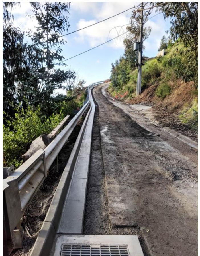
Iluka Extension stabilisation works
