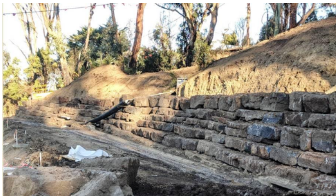
Rock beaching along Separation Creek
