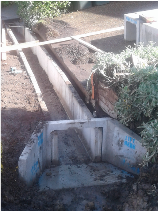
Stormwater system works, Olive Street, Separation Creek
