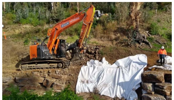
Rock Beaching on Creek Bank taking Shape
