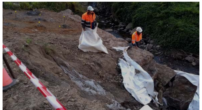
Rock Beaching on Creek Bank taking Shape
