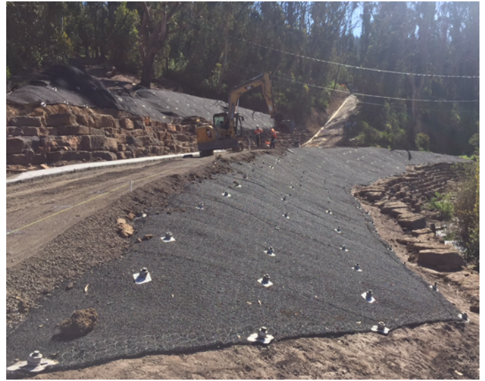
Stanway Drive stabilisation works are nearing completion
