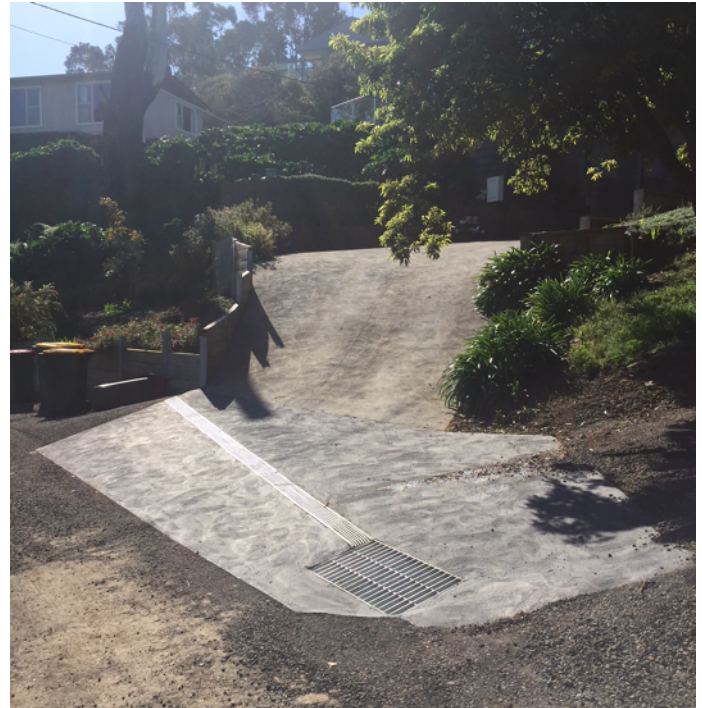
Work is progressing well on driveway culverts across Wye River and Separation Creek
