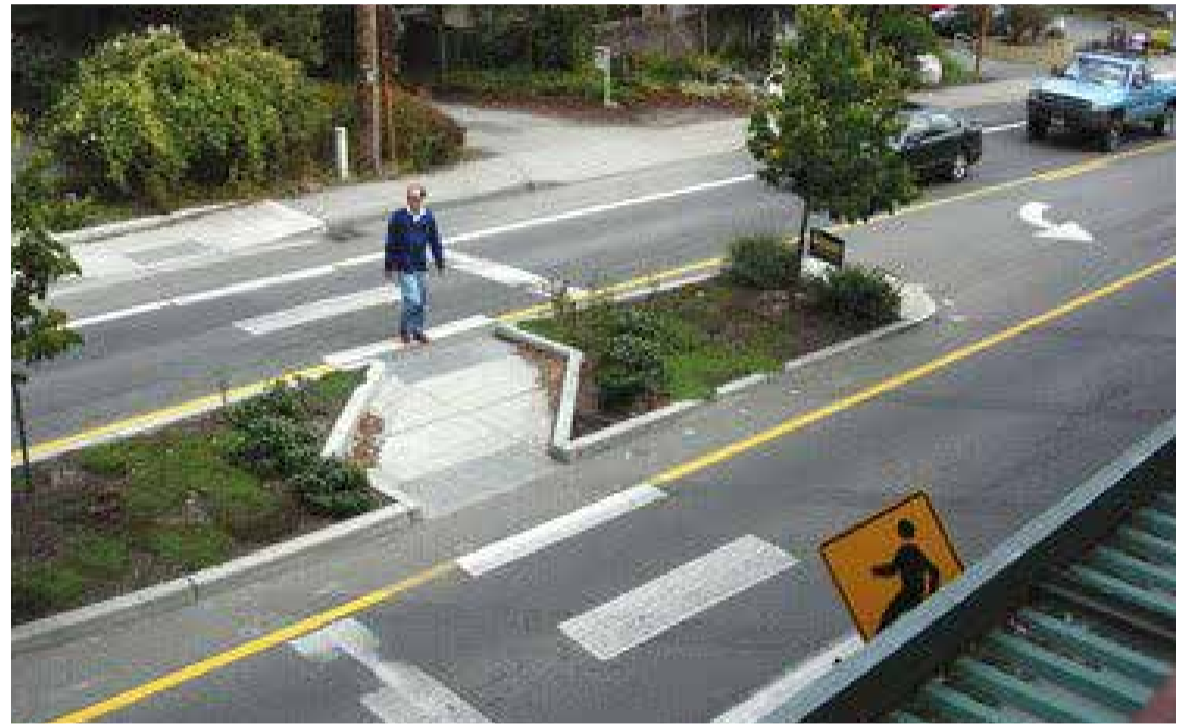
C.1 Pedestrian refuge to reduce the crossing distance across Collingwood Street.
