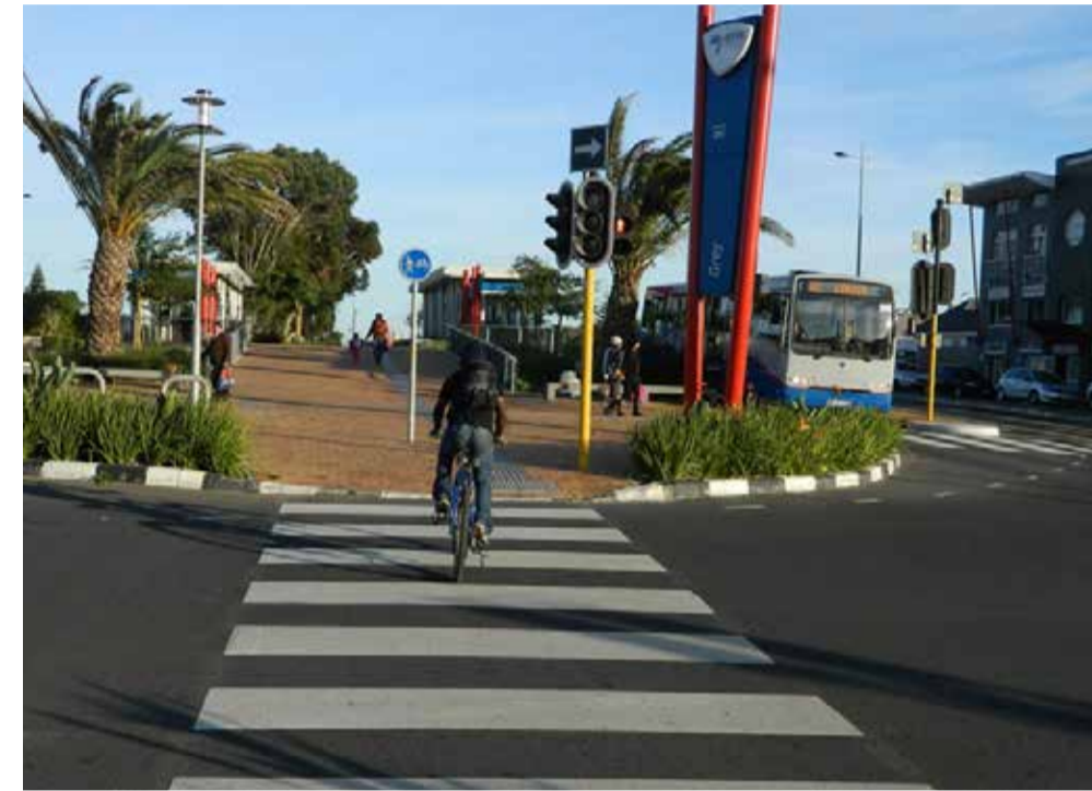
C.3 Kerb outstands and zebra crossing to prioritise pedestrian access.
