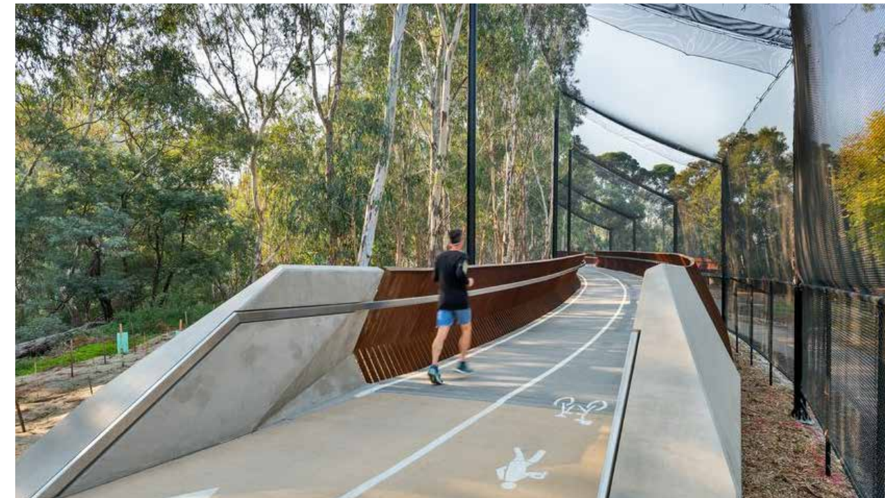
H.8 Shared path with netting to provide protection from balls from adjacent golf course.
