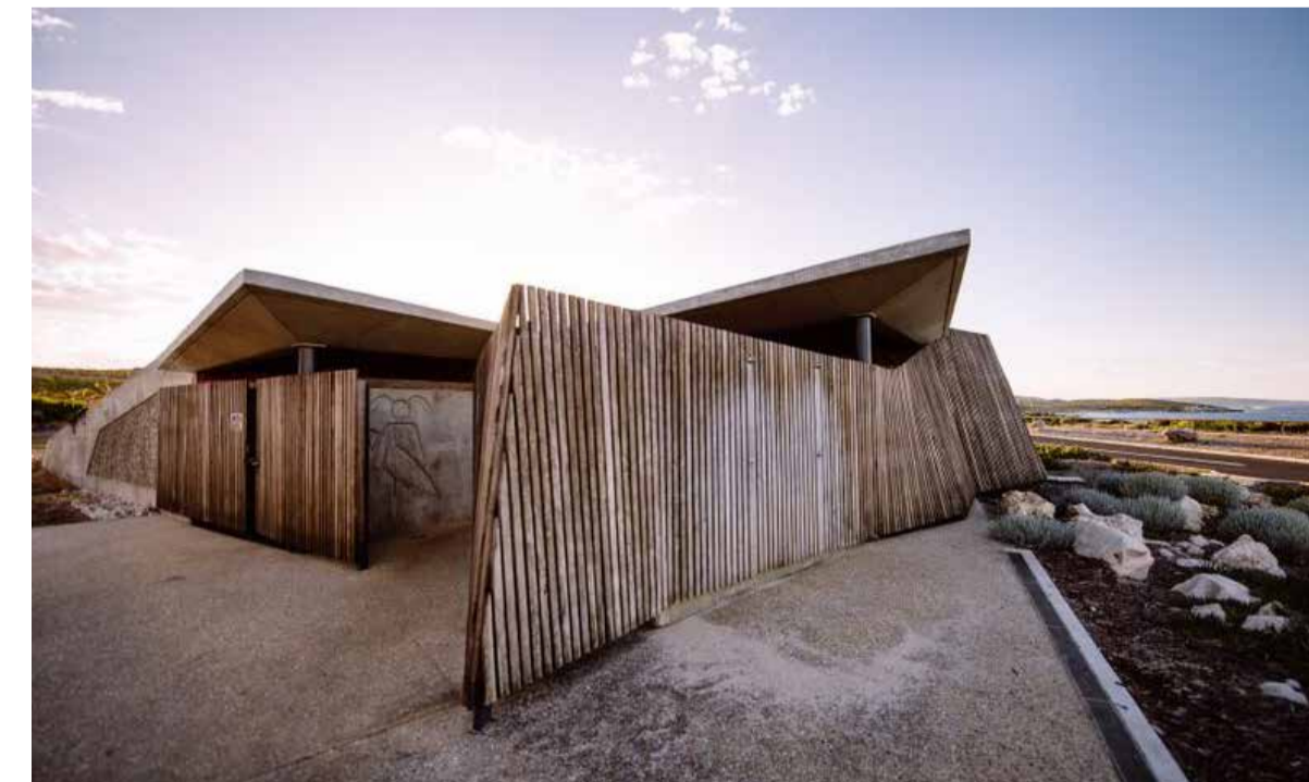
A.13 Well designed public toilets, reflecting the coastal character of the foreshore.
