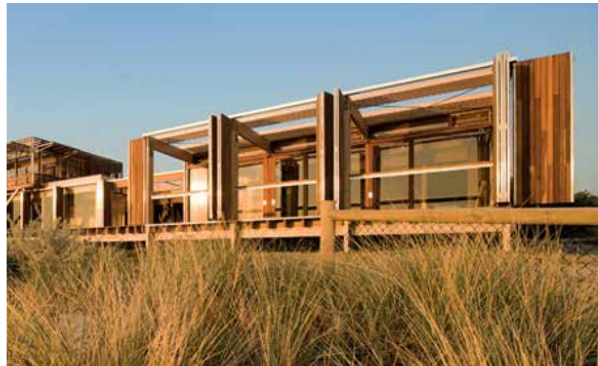
S.1 Contemporary built form orientated to maximise views to the water.
