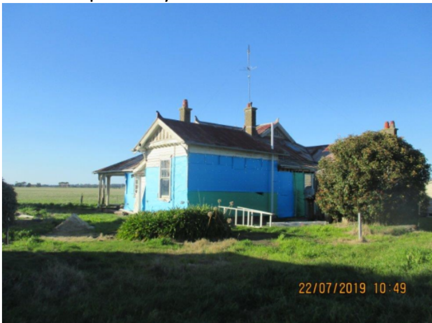
Officer site inspection - July 2019
