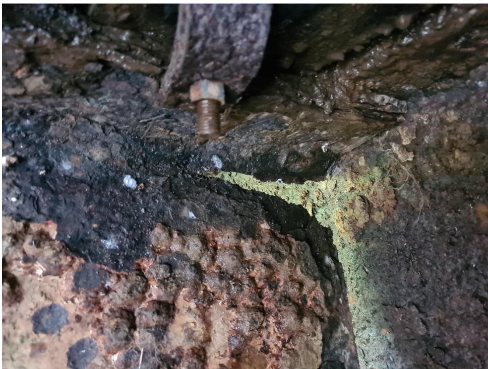
Image 2: Howells Access Bridge over Skenes Creek, heavy corrosion of beams
