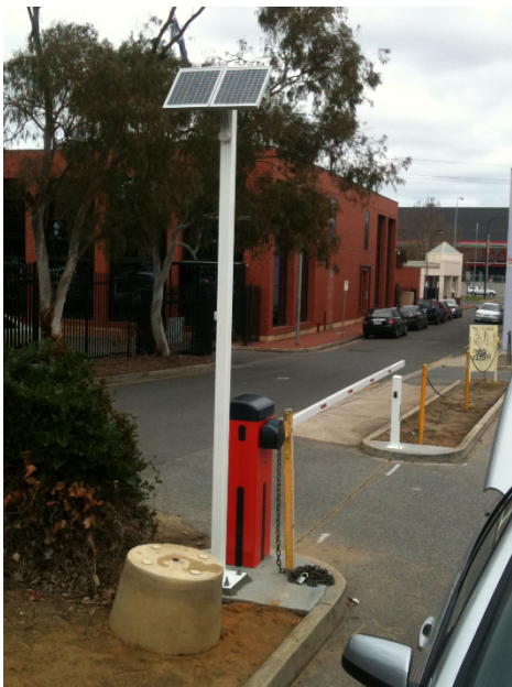
Image 1: An example of a solar powered boom gate
