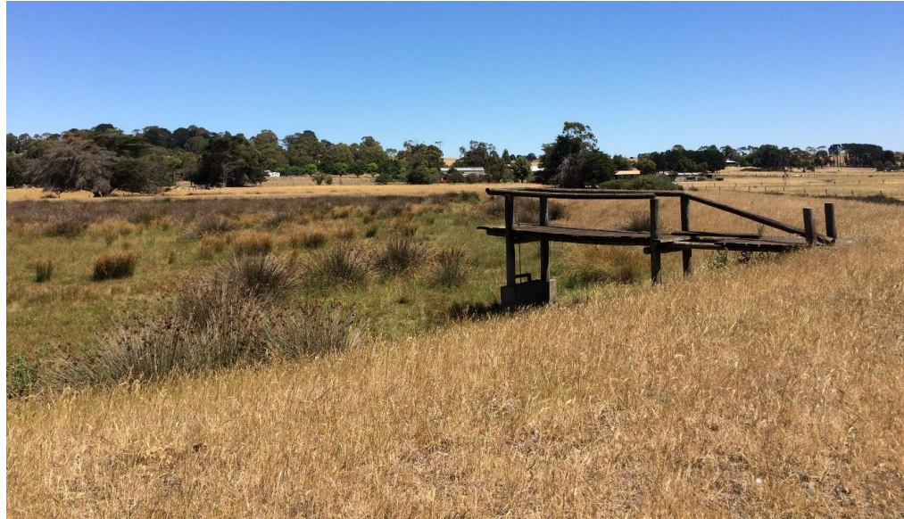
Figure 2.3 Retarding basin Outlet from the top of the embankment
