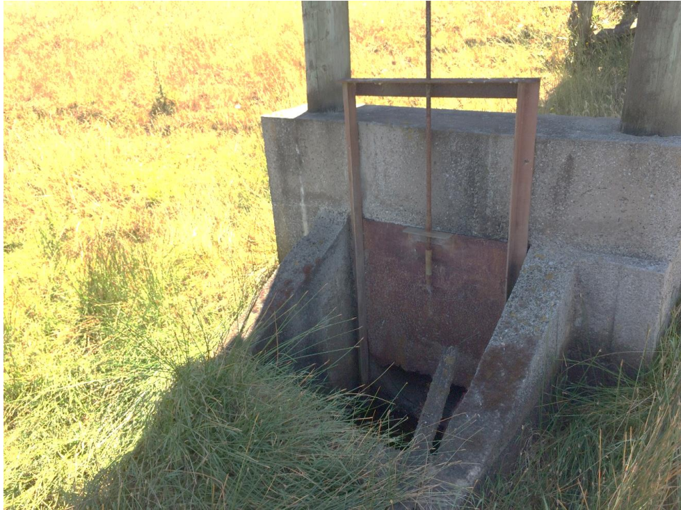
Figure 2.5 Outlet of retaining basin
