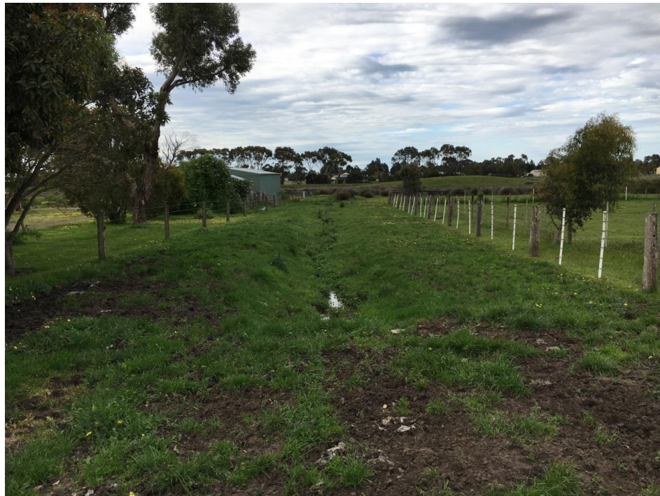
Figure 2.7 Swale into basin from Ballagh Street
