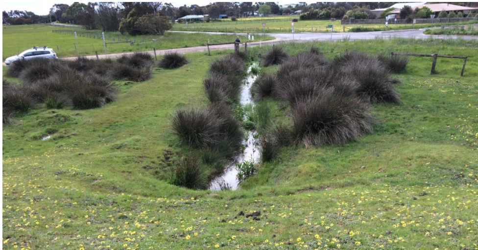
Figure 2.6 Outlet of retaining basin facing downstream
