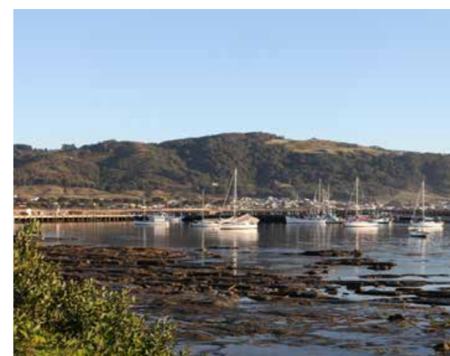
Image 62. Existing berths located along the inner breakwater at Apollo Bay.
