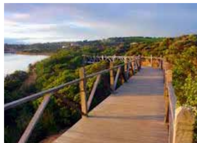
Image 32. Simple timber pedestrian boardwalk allowing access along waters edge.
