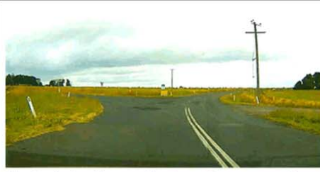
Photo 2: Looking north along Rossmoyne Road over the intersection, Kellys Lane is at left of picture and Boylans Road is at right. Note the fast left turn into Kellys Lane.
