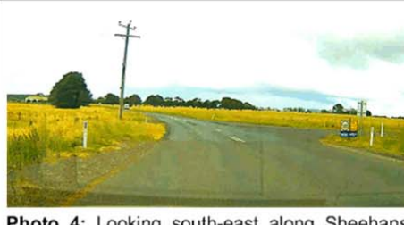
Photo 4: Looking south-east along Sheehans Road over the intersection. Kellys Lane is at right of picture and Boylans Road is at left. Note the hazardous power pole at left of carriageway.
