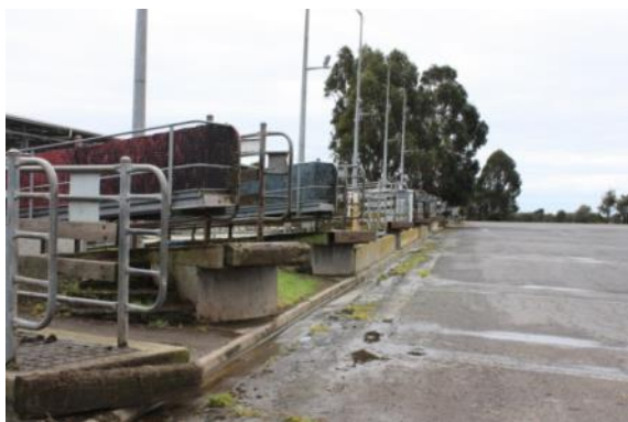
Front Loading Ramps: Note failed bitumen holding rain water
