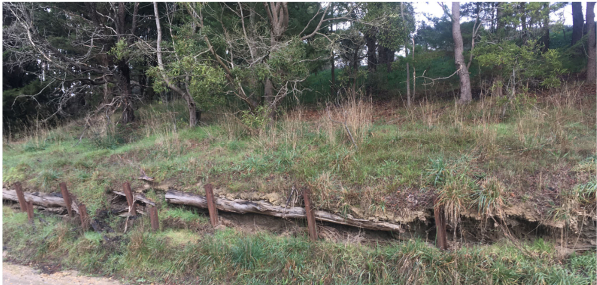
Photo 32: Failed retaining wall at toe of road cutting in Pxvb materials, Pennyroyal Station Road. Natural slope about 8 degrees, modified slope about 12 degrees.
