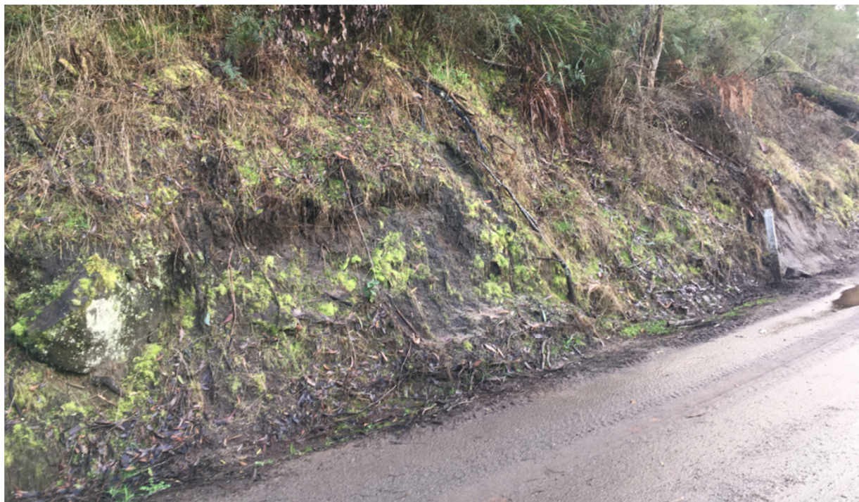
Photo 16: Inferred drape of Pww sand (grey sand) over Koe materials exposed in a road cutting on the RWC Pumping Station Track, Carlisle River. The mapped surface geology in this area is Pww.
