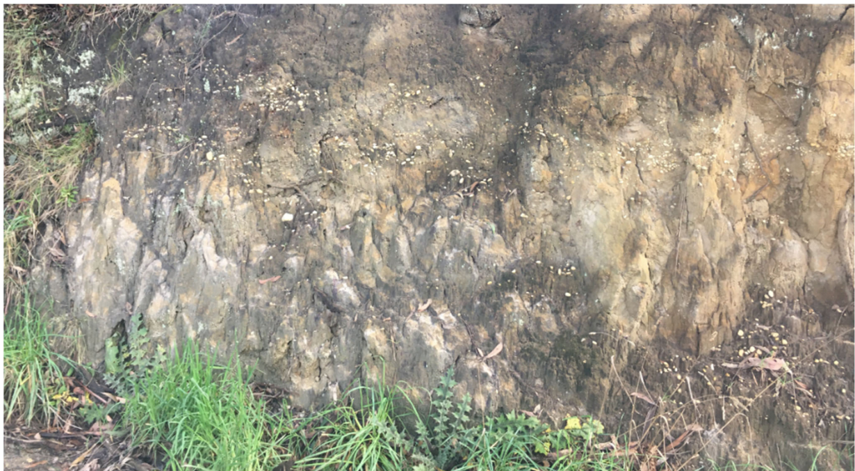
Photo 13: Pwm materials exposed in a road cutting on Lavers Hill-Cobden Road near its intersection with the Gellibrand River Road.
