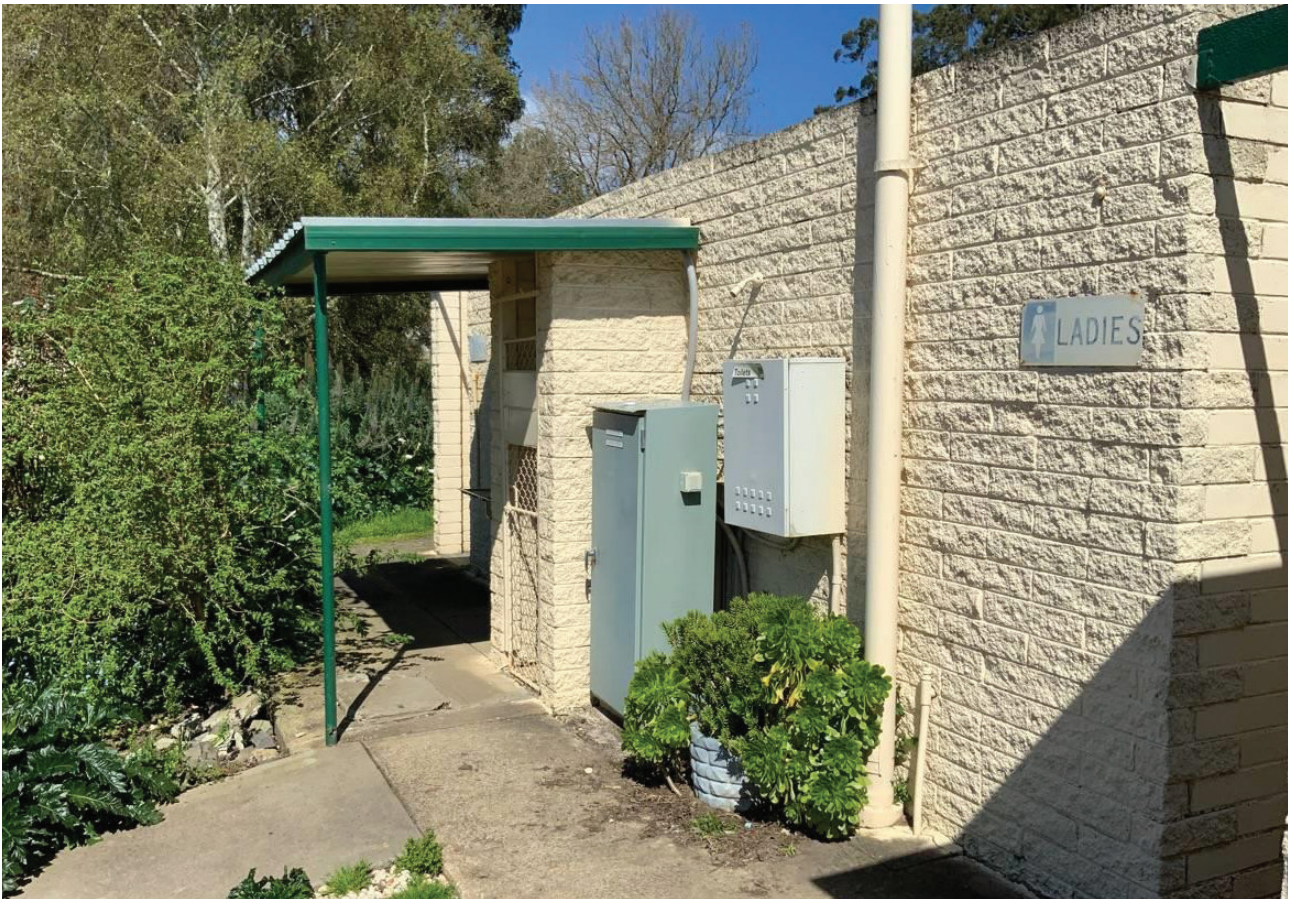
Figure 3: Forrest Caravan Park Public Toilets
