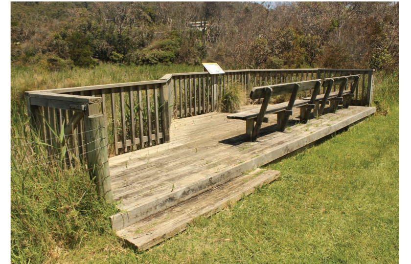
Existing deck overlooking wetland to retain, likely to inform material and style of proposed furniture/ finishes.
