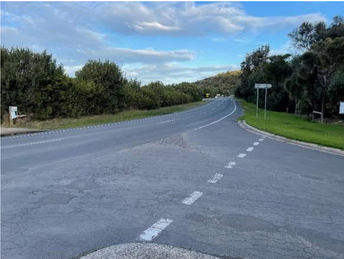
Photograph 5: Hawdon Avenue – at Great Ocean Road view to south.
