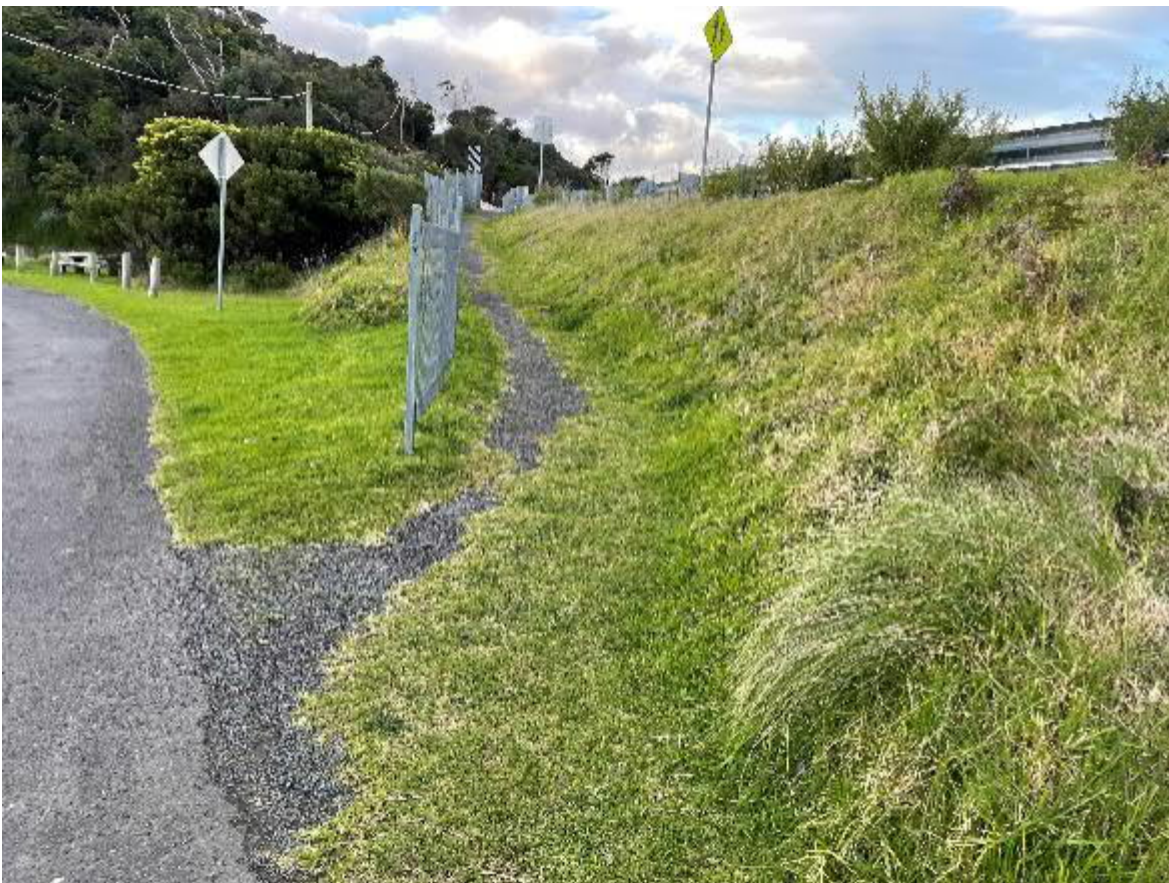
Photograph 10: Great Ocean Road service road – view to Kennett River Bridge.
