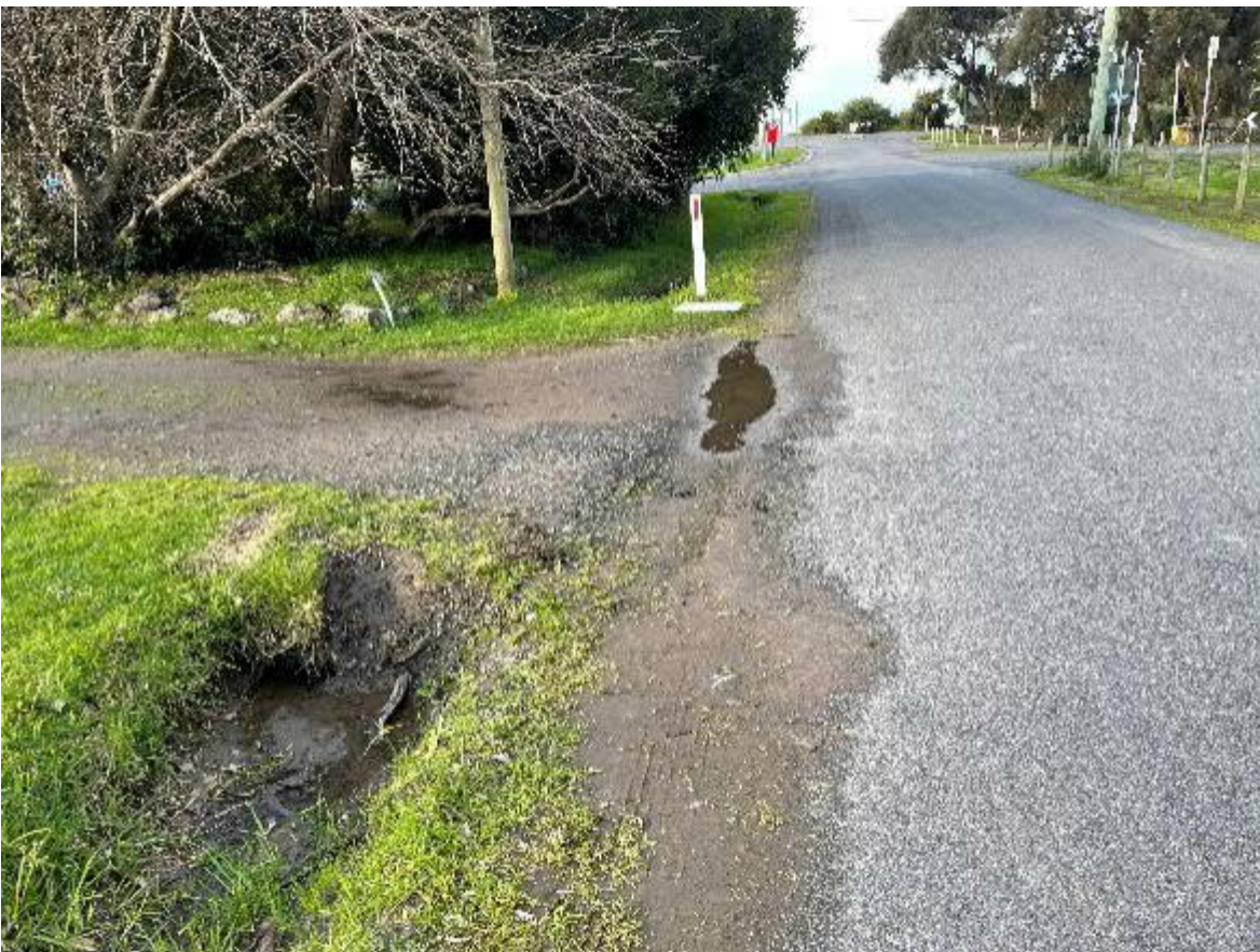
Photograph 6: Hawdon Avenue – west of Grey River Road view to east.
