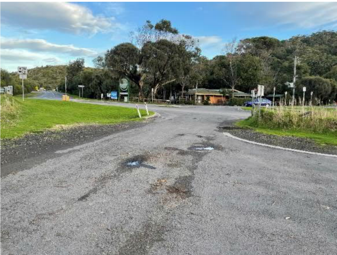
Photograph 4: Great Ocean Road service road – north of Hawdon Avenue view to south.
