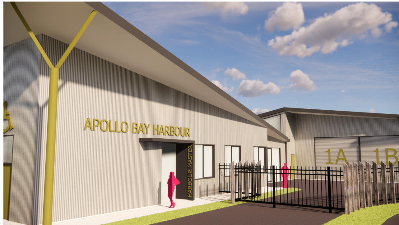
VIEW OF BUILDING ENTRY
