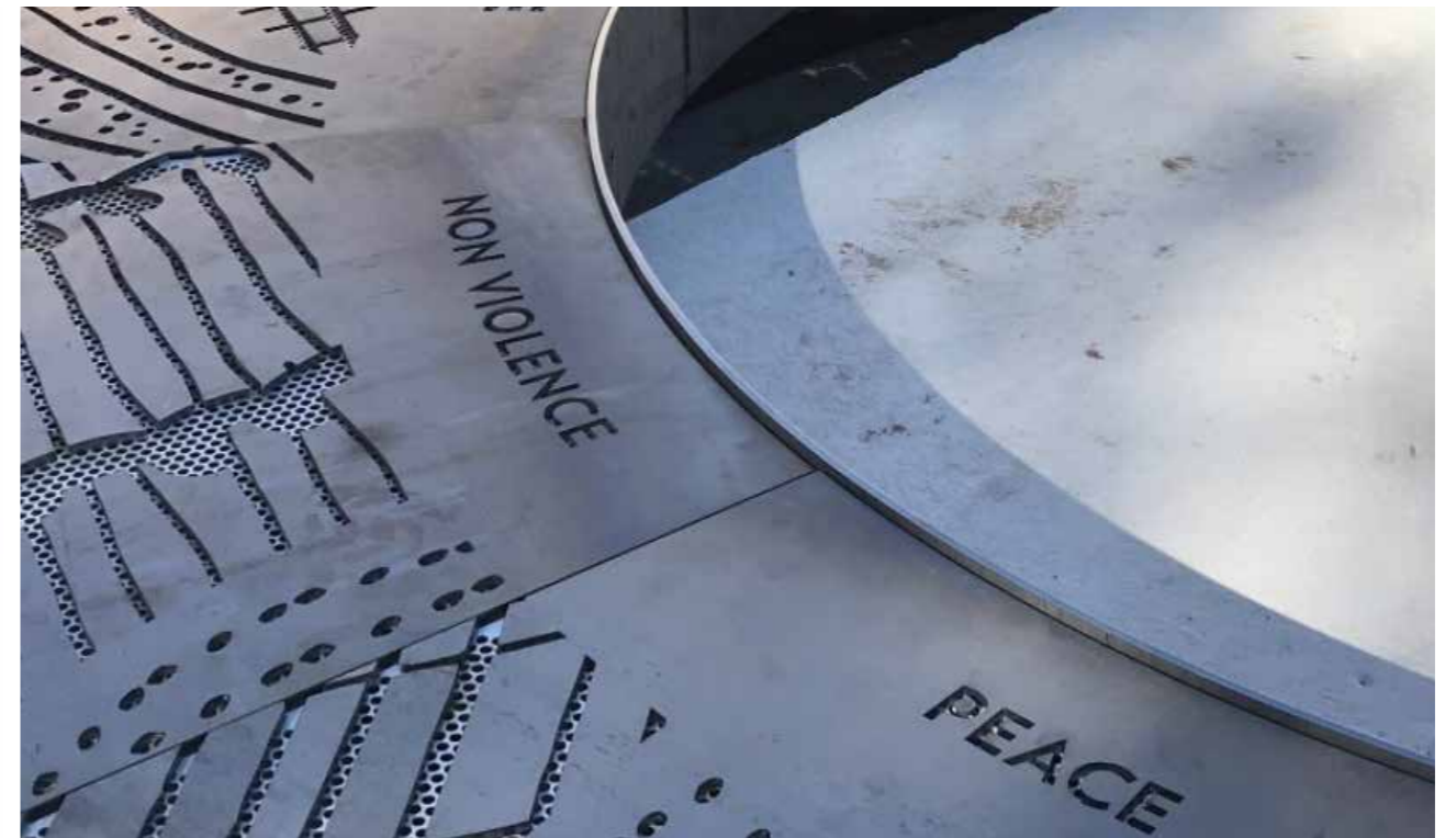
Example of historical information laser cut into brass plate with perforated back.
