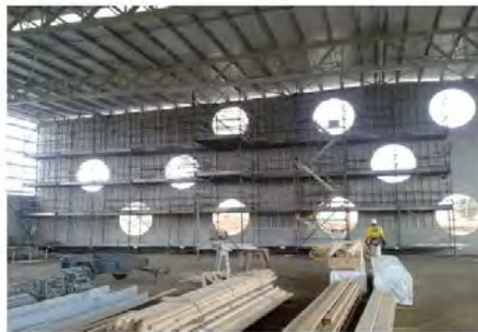
Wall battening to stadium in preparation for wall linings
