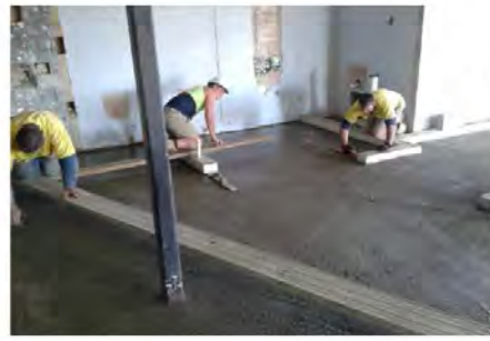
Concrete screeding in wet change rooms
