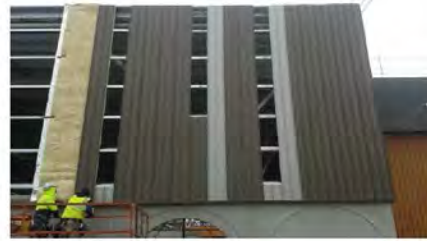
Installation of external cladding to stadium
