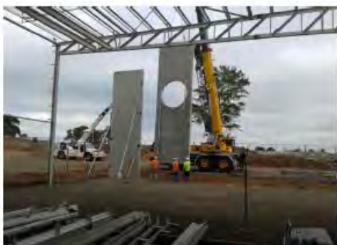
Precast panel erection
