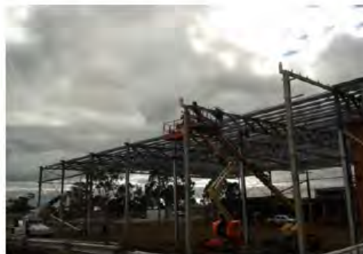
Extension of existing stadium roof trusses
