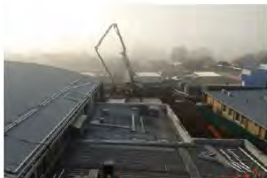
Pouring of plant room floor
