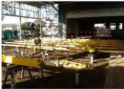
Construction of subfloor to gymnasium
