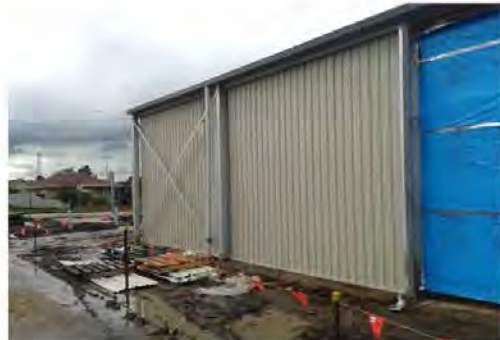
New metal cladding to minor hall
