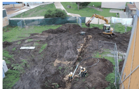
Excavation for new fire service ring main
