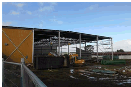
Demolition of existing stadium cladding
