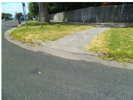
Lips (bullnoses) at Kerb Ramps are difficult to negotiate with Mobility aids
