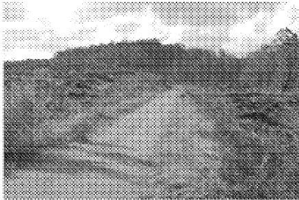
Figure 46: Former railway embankment and cutting, alongside Banool station site. The formation has been compromised by pine plantations and timber harvesting. Looking north. Source: Context 2012
