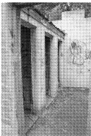
Internal view of 1930's toilet block
