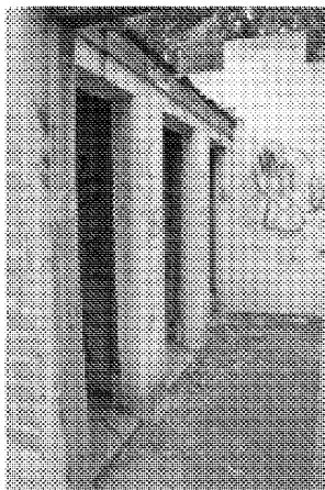
Internal view of 1930's toilet block
