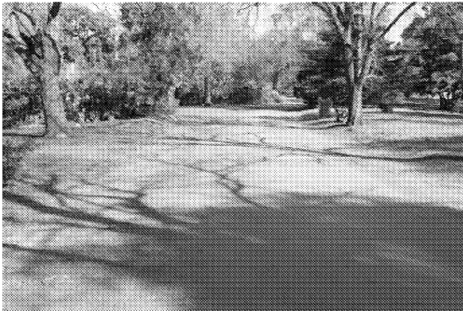
Carriageway within the Colac Botanic Gardens, showing wear pattern and consequent incremental widening of track surface.
