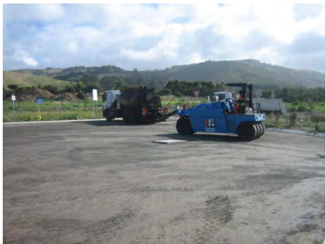
Apollo Bay Transfer Station – Primerseal prior to asphalt
