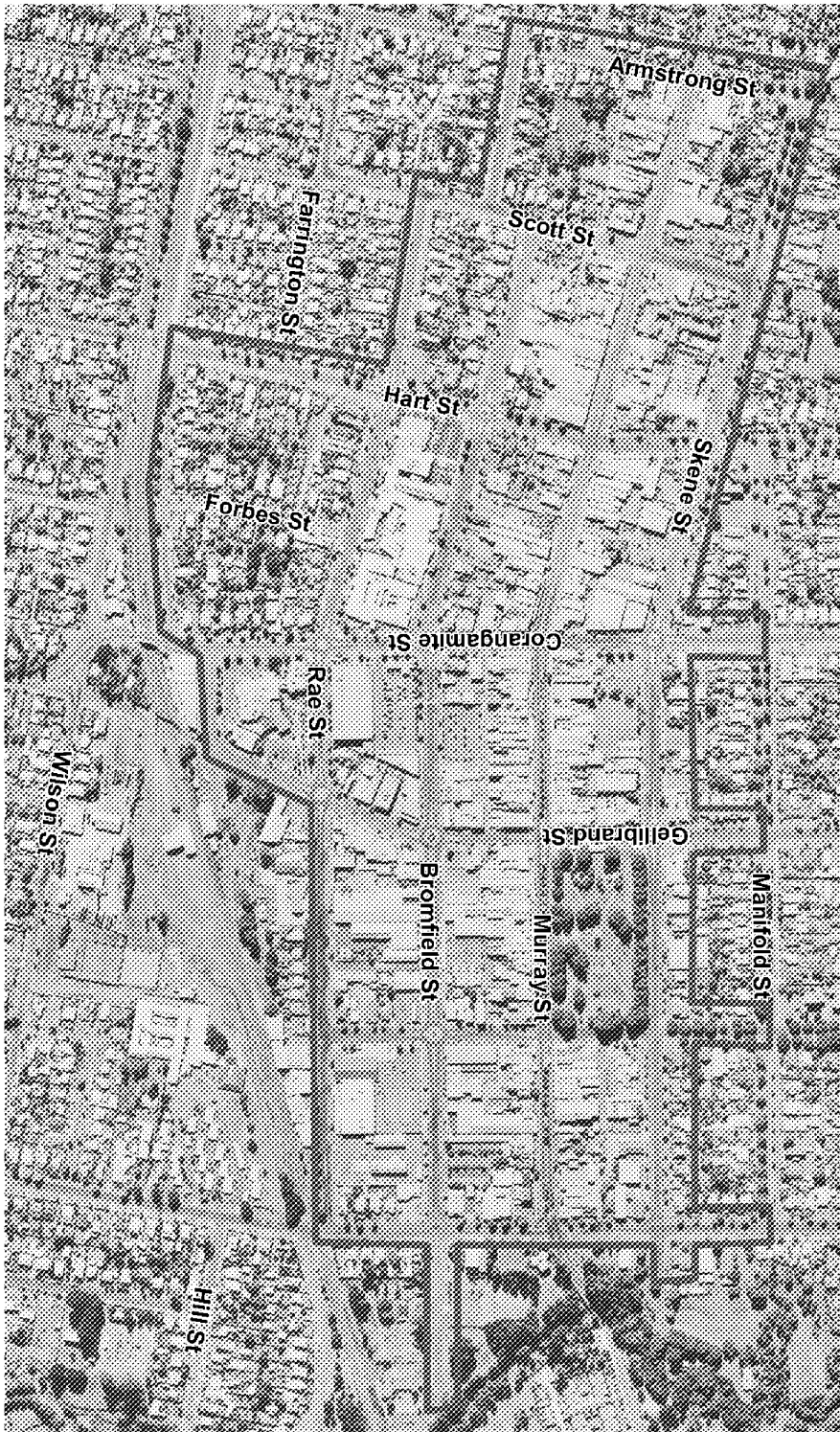
Figure 1.1 : Aerial Photo of Colac Commercial Centre (area bounded by red line)
