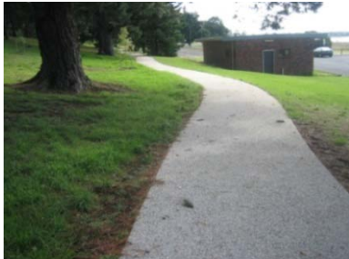
Exposed Aggregate Footpath
