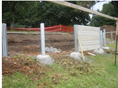
Construction Of Viewing Platform
