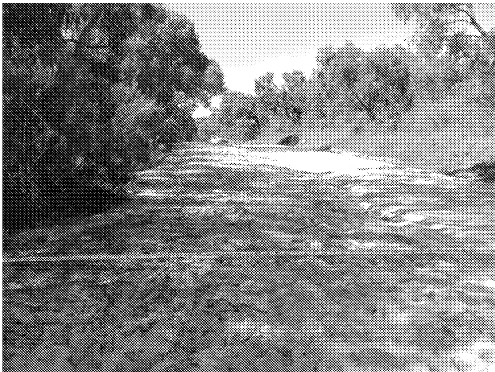
Figure 6. Vegetation removed on east side of Hargreaves Track (5 metre width). Note vegetation removed on west side of track.
