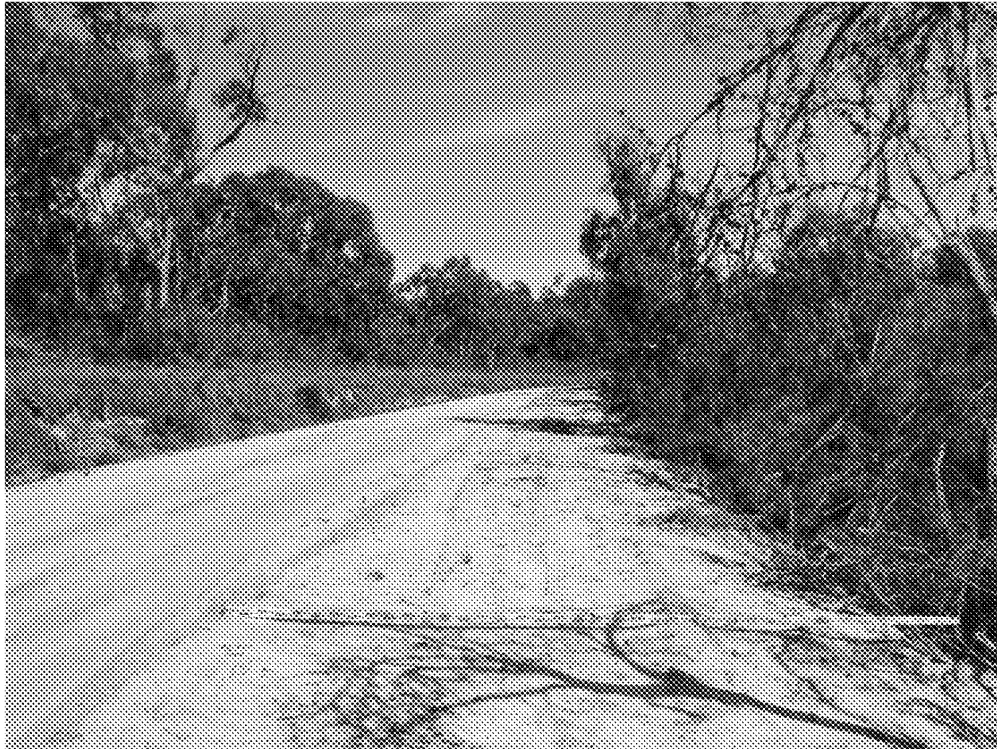
Figure 5. Vegetation removed on east side of Hargreaves Track (4 metre width). Note vegetation removed on west side of track.
