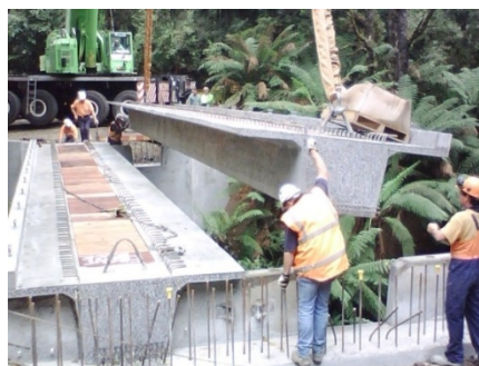
Placing Super T Beams
