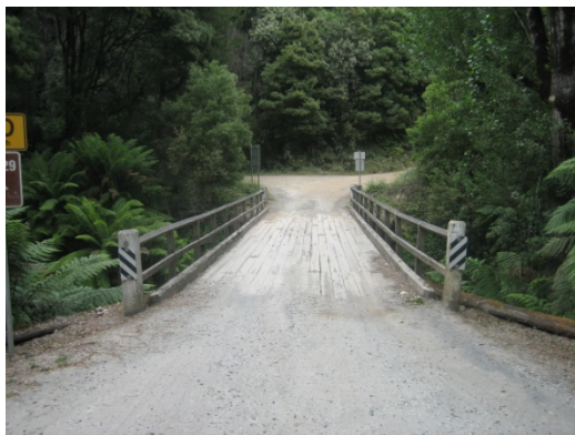
View of existing timber bridge in Binns Road
