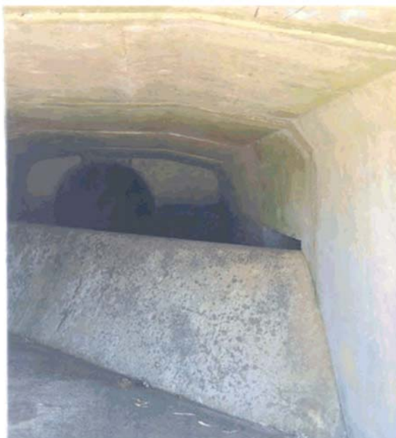
Photo 3 – Low flow diversion to GPT within drainage outlet structure (near intersection of Queens Ave and Armstrong Street)
