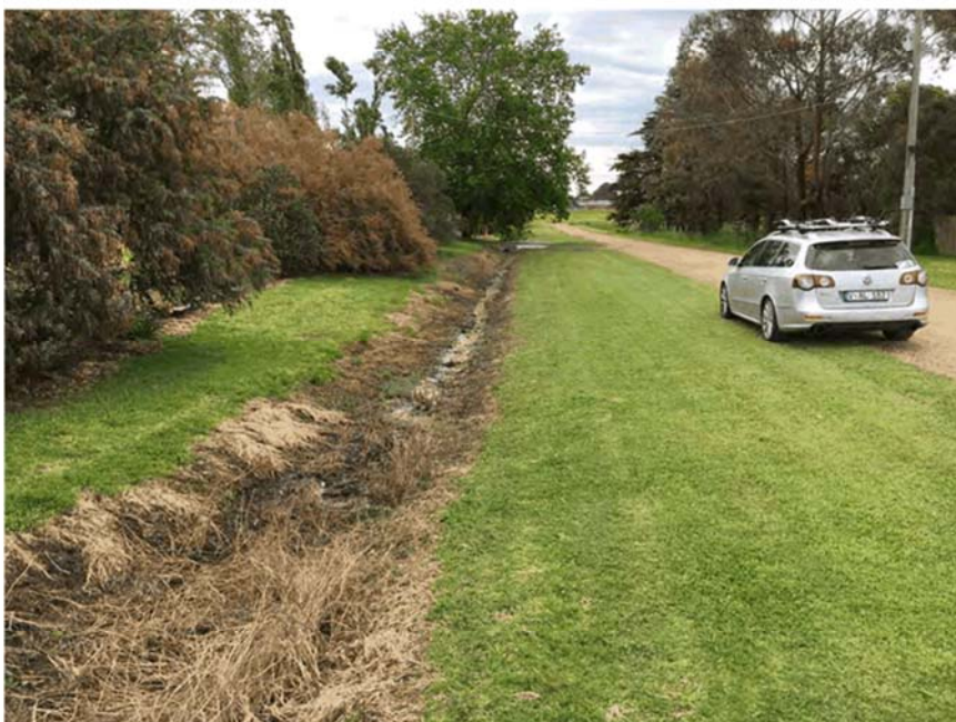
Photo 9 – Drainage swale alongside Ballagh Street
