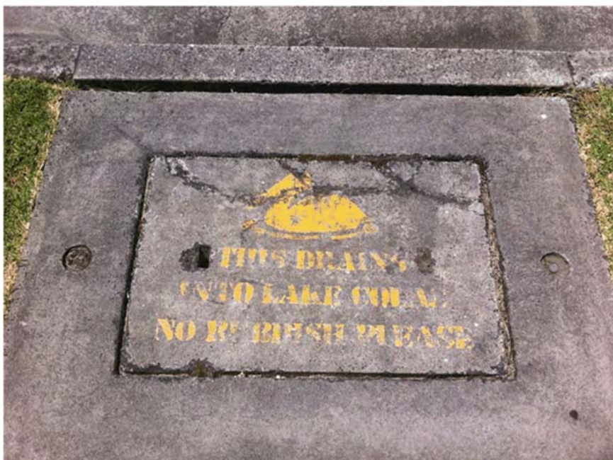
Photo 7 – Stormwater pit lid indicating Lake Colac as outlet to drainage network
