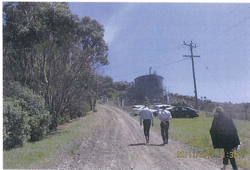
looking west toward tower
