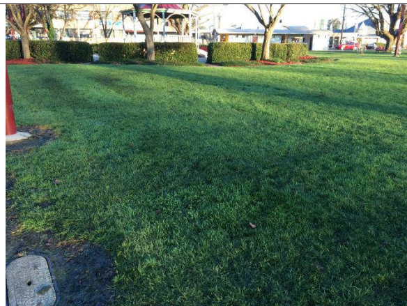
11. Damage from foot traffic around market stall area
