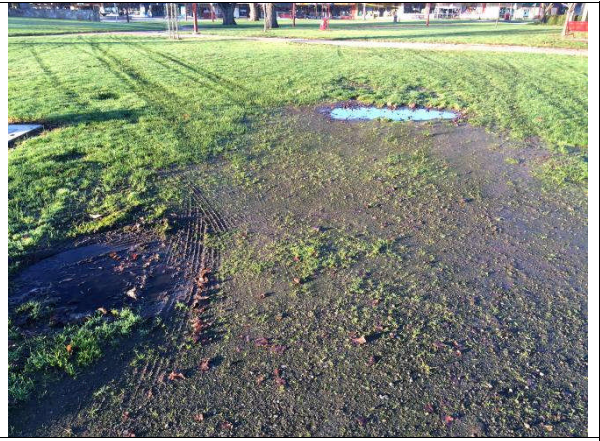
14. North side vehicle access point, showing rutting in lawns as vehicles move off sealed area
