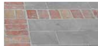
Option 2: Concrete pavers with brick edging
