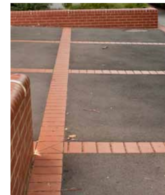
Option 4: Asphalt footpath and brick edging
