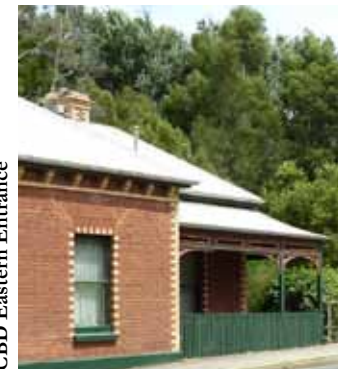
CBD Eastern Entrance
