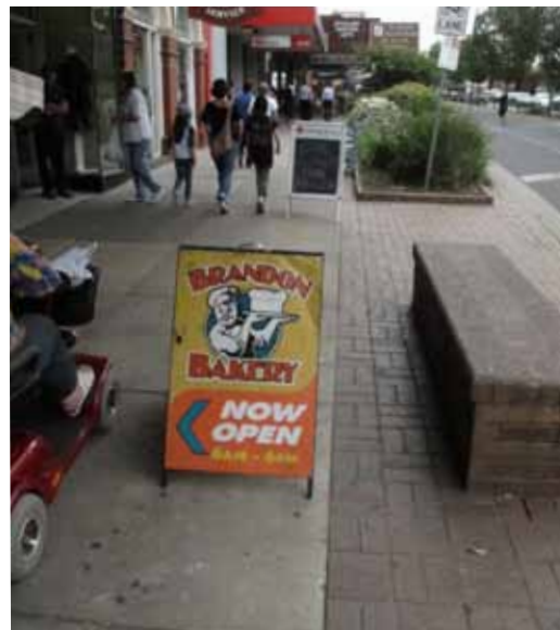
Existing Murray Street pavement in need of refreshment
