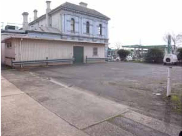
Telephone exchange site where there is potential to improve the side of the former Post Office, which needs restoration and painting
