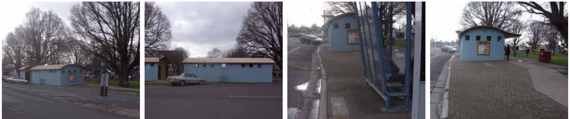
Toilet block facility is outdated and forms an unattractive edge to Memorial Square
