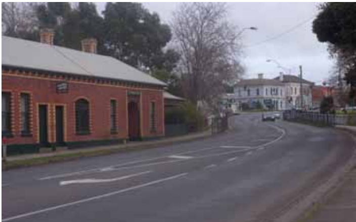
View along Princes Highway to Barongarook Creek bridge with the CBD, corner of the telephone exchange site and notable historic buildings
