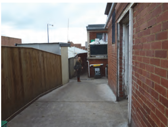
Existing pedestrian laneway situated between 79 and 81 Great Ocean Road
