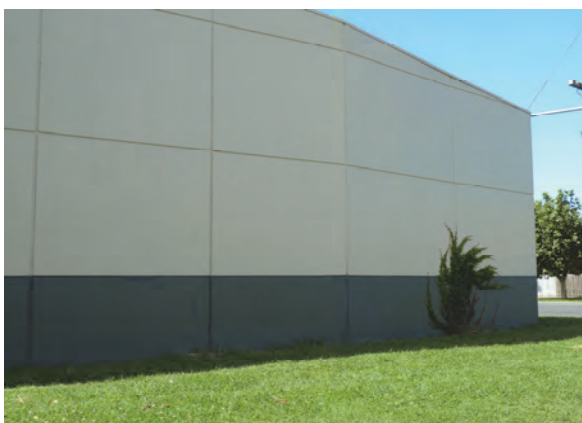
Existing blank wall fronting Pascoe Street
