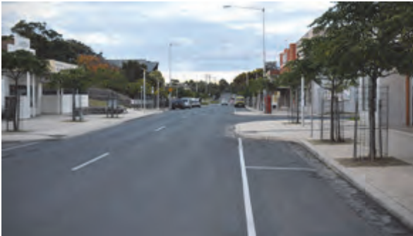
Kerb outstands, parking bays and new street tree planting have improved the amenity and function of Hitchcock Avenue, Barwon Heads
