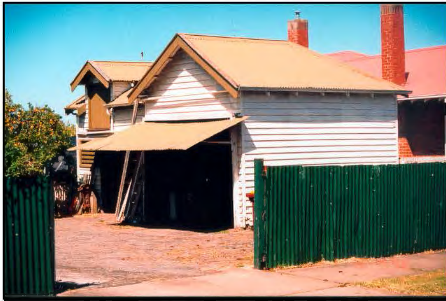
Timber Stables, rear of 16 Fyans Street Colac.
