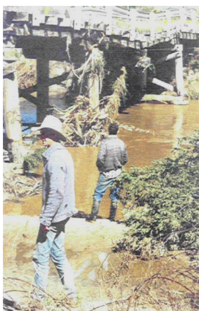
Bridge damage after a flood
