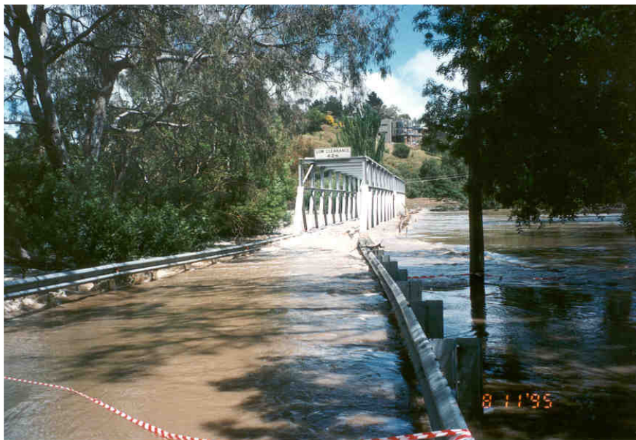
Barwon River at Queens Park Bridge Geelong in November 1995.
