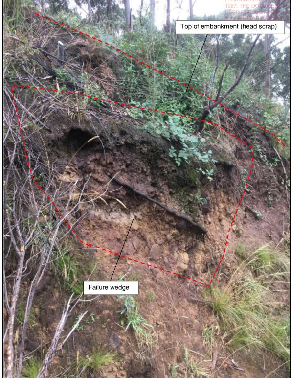
Existing site cut (wide view) top of site, note small failure wedge at top of embankment
