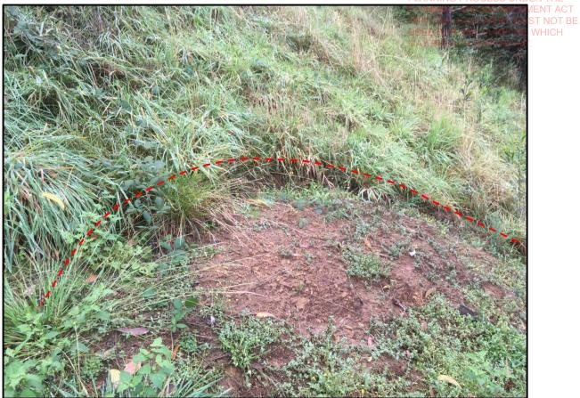
Existing site. Fill/recent spoil placement., note scarp outline, indicating soil movement / possible slope instability
