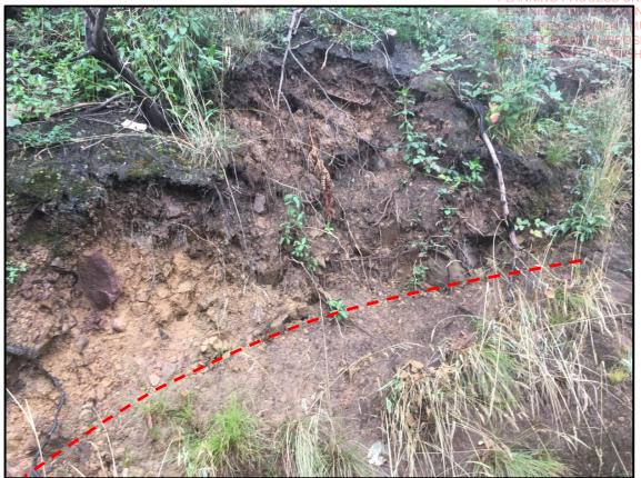
Existing site cut, top of site, note recent failure at top of embankment
