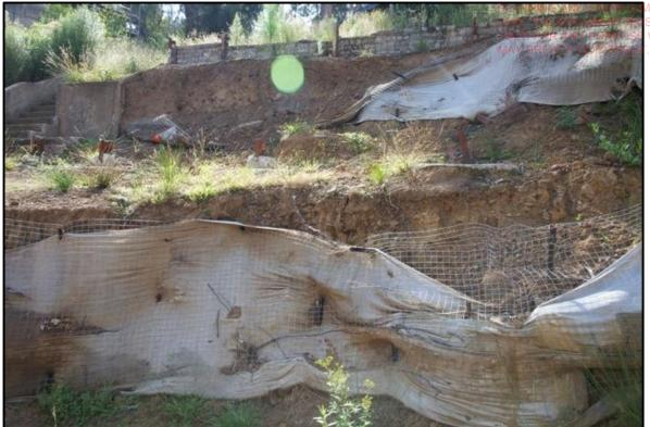
Adjacent site No. 42 Riverside Drive-low strength rock (possible colluvium in cutting)
