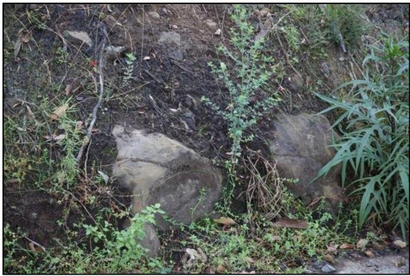
Riverside Drive cutting, displaced boulder size rocks at base of road cutting
