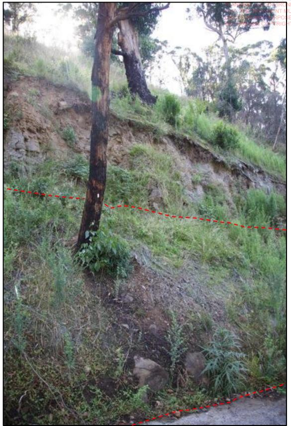
Existing site cut along Riverside Drive, note failure wedge and uneven tree alignment indicating previous slope movement-photo 2
