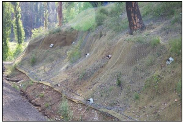
Riverside Drive-recent remedial works including geo-mesh and rock bolting
