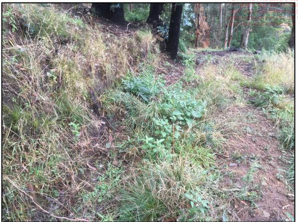
Adjacent site (north). Note existing drain and poorly graded drainage
