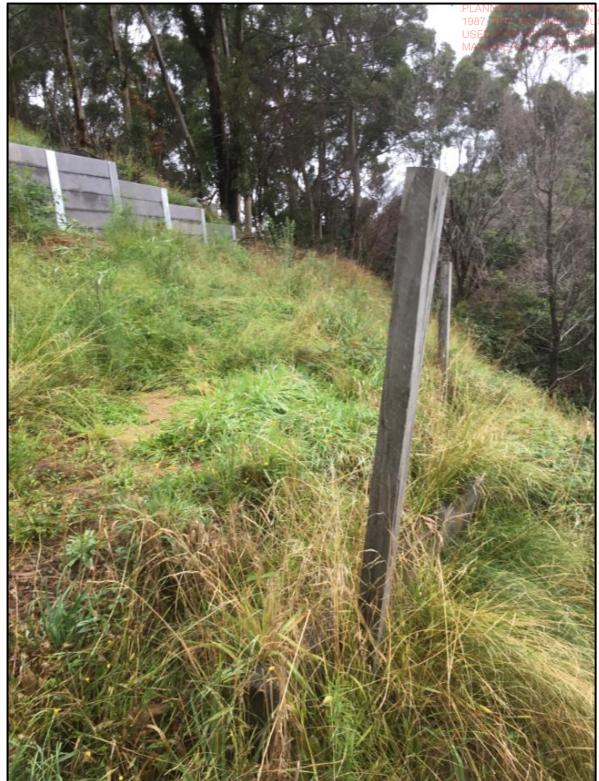
North east view: existing site, note overturning retaining structure
