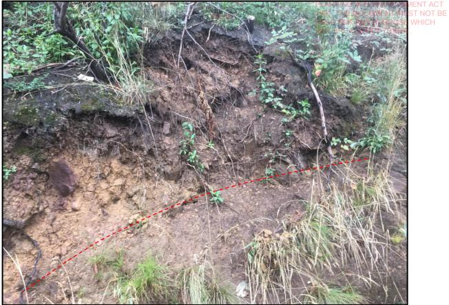
Existing site cut, top of site, note recent failure at top of embankment
