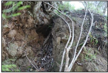
Riverside Drive road cutting, distressed face, imminent small failure-detail
