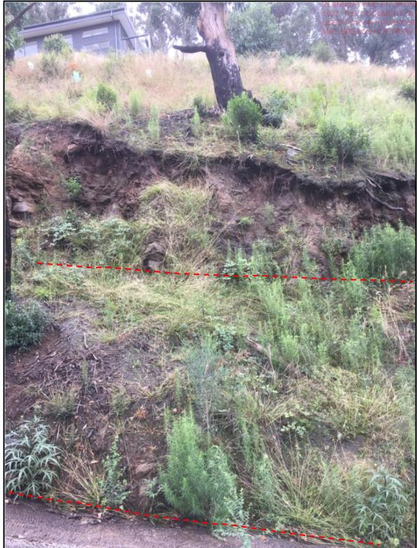
Existing site cut, bottom of site along Riverside Drive, note failure wedge-photo 1
