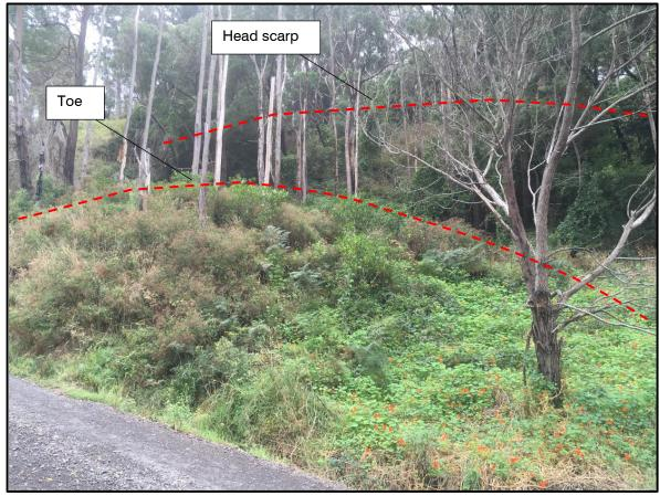
North west view from Riverside Drive: adjacent site, large previous landslide scarp and toe (note toe extends south past Riverside Drive
