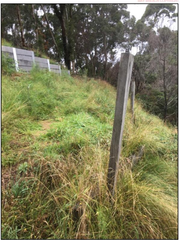
North east view: existing site, note overturning retaining structure
