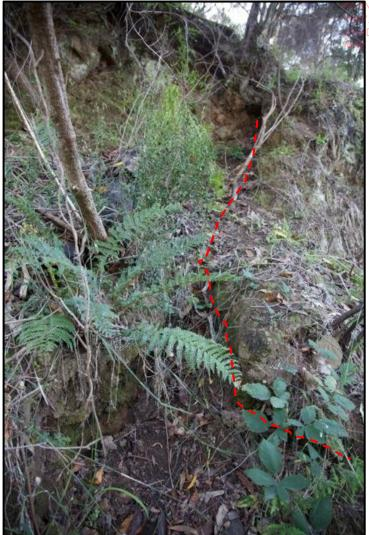
Riverside Drive road cutting, distressed face, imminent small failure
