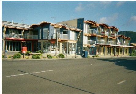
Gateway development: Good combination of modern practice and traditional materials and style.
