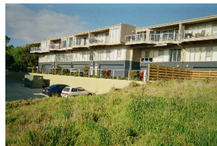
Units at Wild Dog development: Very unsympathetic materials, crude building form with overbearing straight skyline.
