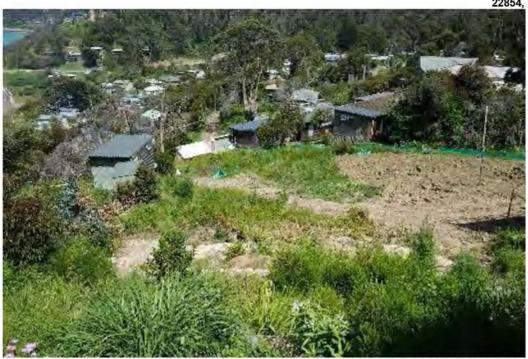
Photo 1 Disposal field looking south west with uncontrolled FILL and incorrect storm water drain construction at the time of inspection. .
