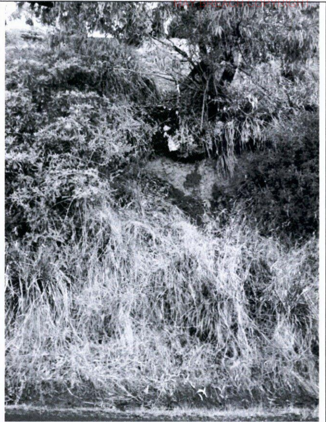
Photo 6: View from Morley Avenue. Groundwater seeps and tree undermined by slumping in cutting.
