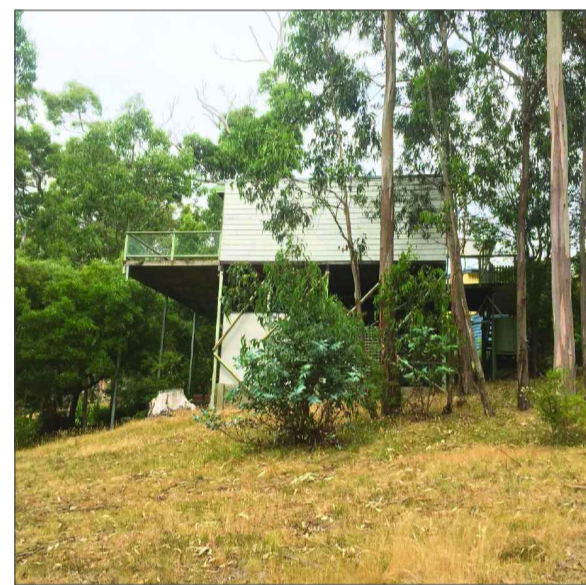
SINGLE STOREY DWELLING ELEVATED HIGH ON STILTS WITH PROTRUDING BALCONY.
