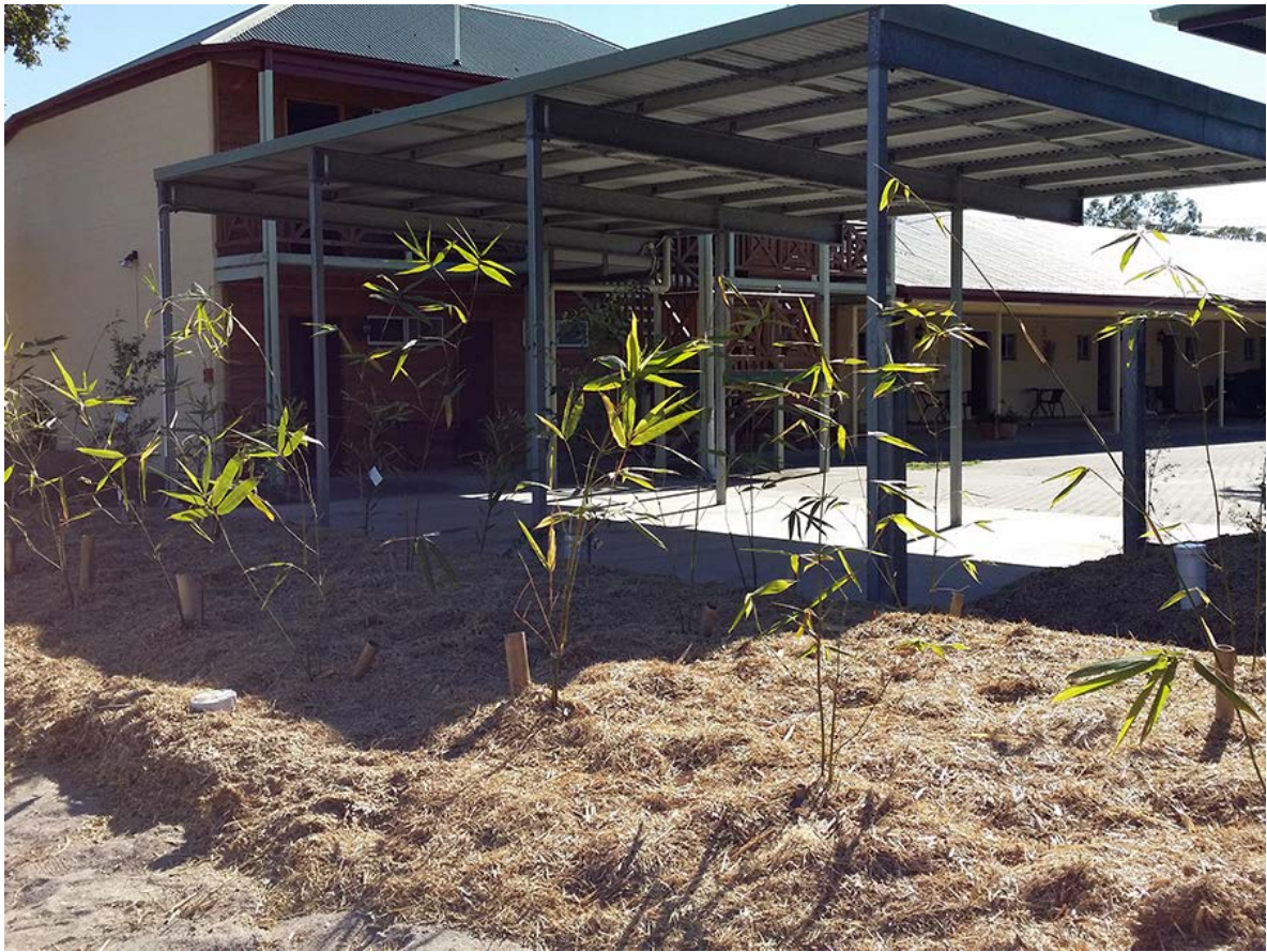
TYPICAL GROUND LEVEL SYSTEM JUST AFTER INSTALLATION
